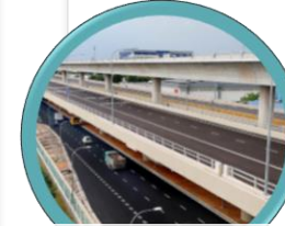
Viaducts | MRT tracks | HSR
